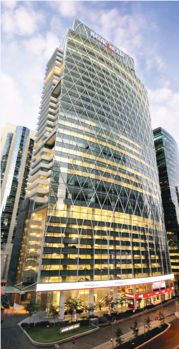
Menara Bank Islam – New Iconic Building at the Heart of KL City Centre
